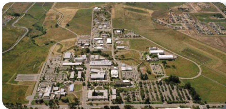
Figure 3.1 SNL/CA Campus, Looking South
